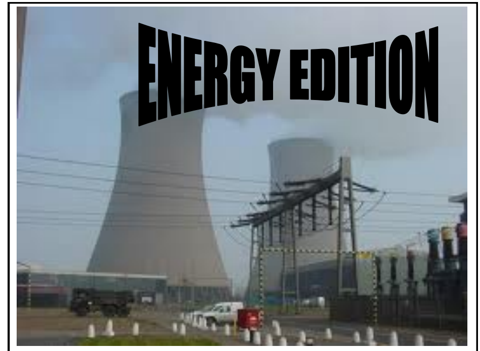
West Burton Power Station
